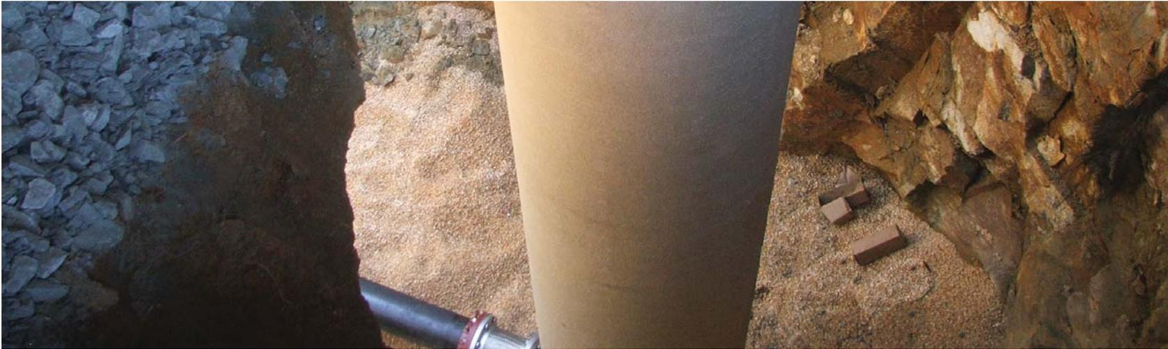
Containment Solutions' vertical pump vault and tank meets the requirements of NFPA 22 for the storage of fire protection water. The fiberglass pump vault can be installed along with a Flowtite® fiberglass tank to complete an underground fire protection storage system. This installation method allows 100% of the tank volume to be accessible.
