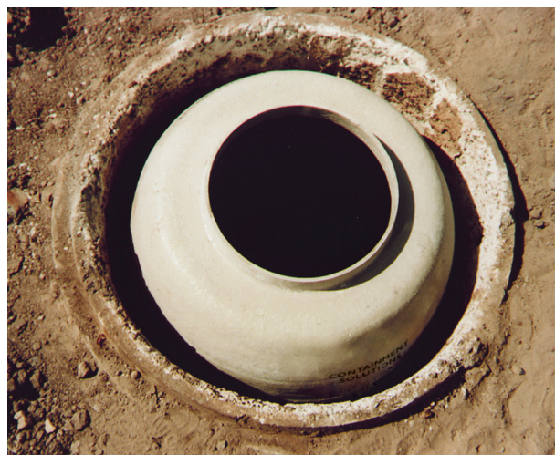
Rehabilitation manholes work independent from the corroded existing manhole.
